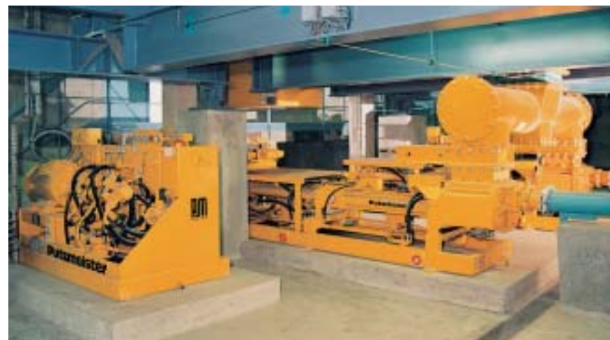
2 high-density solids pumps KOS 1030 to charge sewage sludge into the garbage incinerator in Dinan, France
