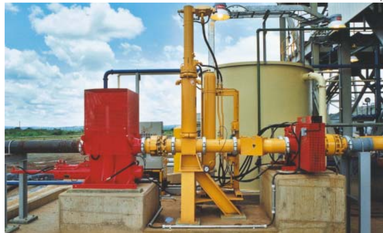
ZX 200 pig gate, HPD 200/750 high pressure damping vessel and DVH 412 transfer tube
